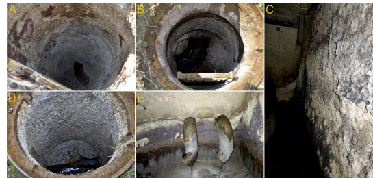
Fig. 3 – Photos of MIC in sewage facilities [17], Photos (A), (B), (D) are taken from the manhole of sewage pipes; Photos (C) and (E) are taken from wastewater catchment basins.
